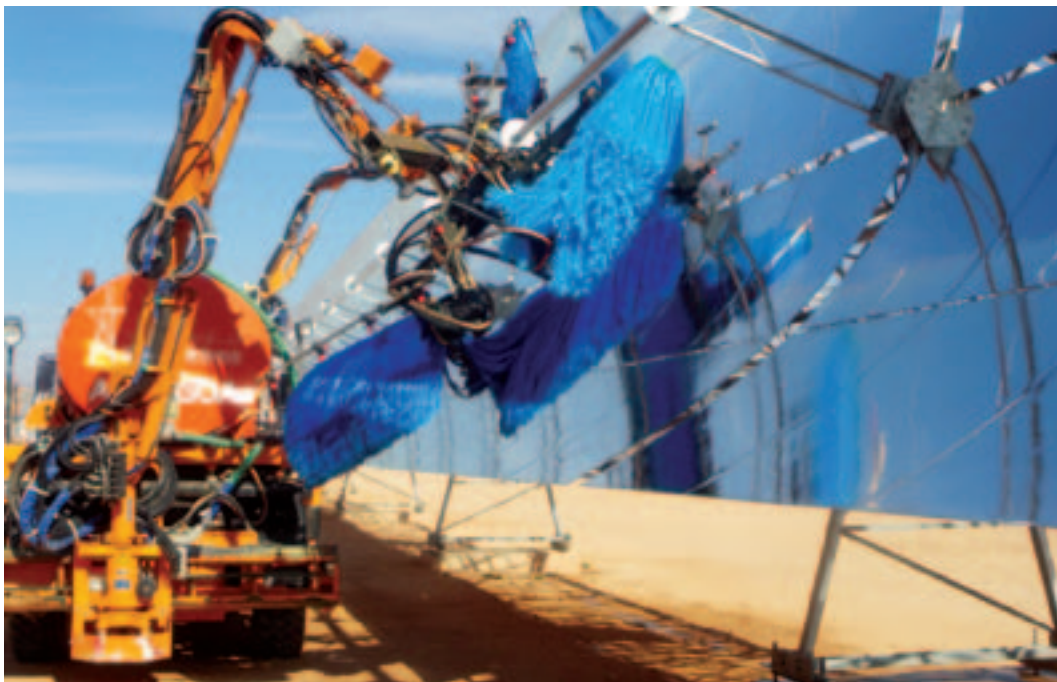
Photo 8.2 Cleaning of parabolic troughs at Ain Beni Mathar (Morocco)
