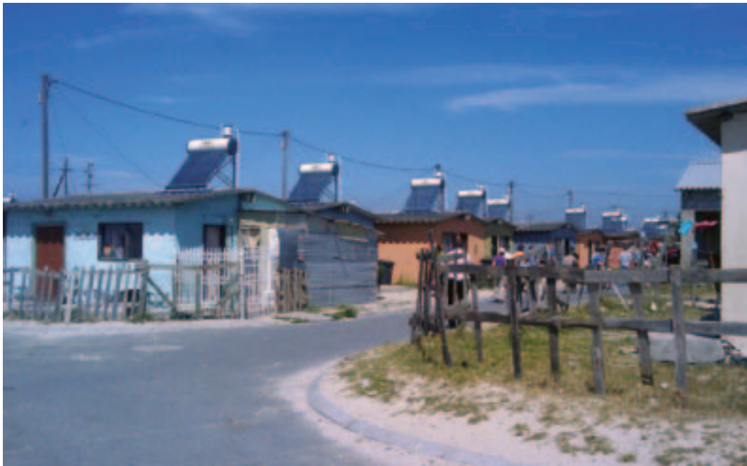
Photo 4.3 Solar water heaters in South Africa
