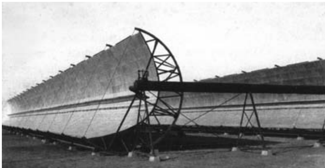
Photo 8.1 Shuman’s concentrating solar thermal plant in Maadi, Egypt, 1913
