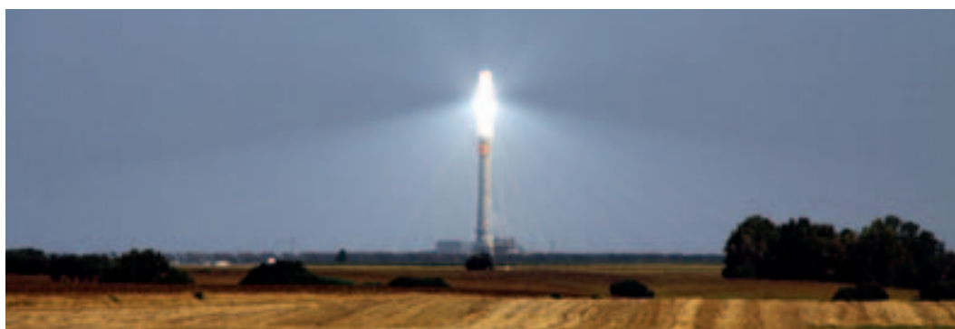
Photo 3.1 The Gemasolar power tower near Sevilla (Spain)
