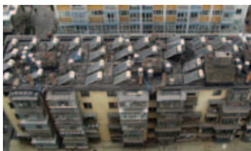
Photo 4.2 Solar water heaters in Kunming, China
