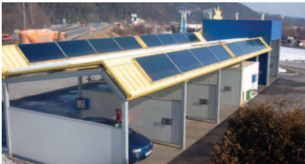
Photo 5.1 Solar water heaters can be used in service areas
