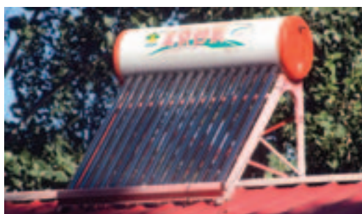
Photo 4.1 Chinese thermo-siphon solar water heater
