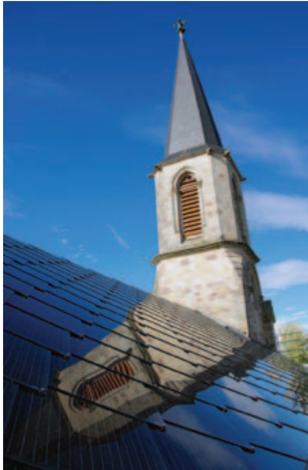
Photo 4.5 Manspach church (Alsace, France) renovated using photovoltaic tiles
